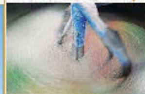
2 to 3 minutes Continuously Concrete Mixing 5
