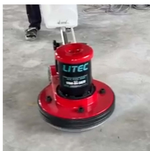
CEMENT SURFACE PREP
